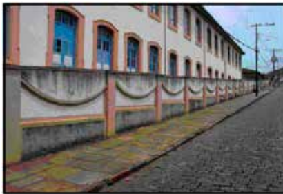
Figure 2: Curves on the wall of the school
